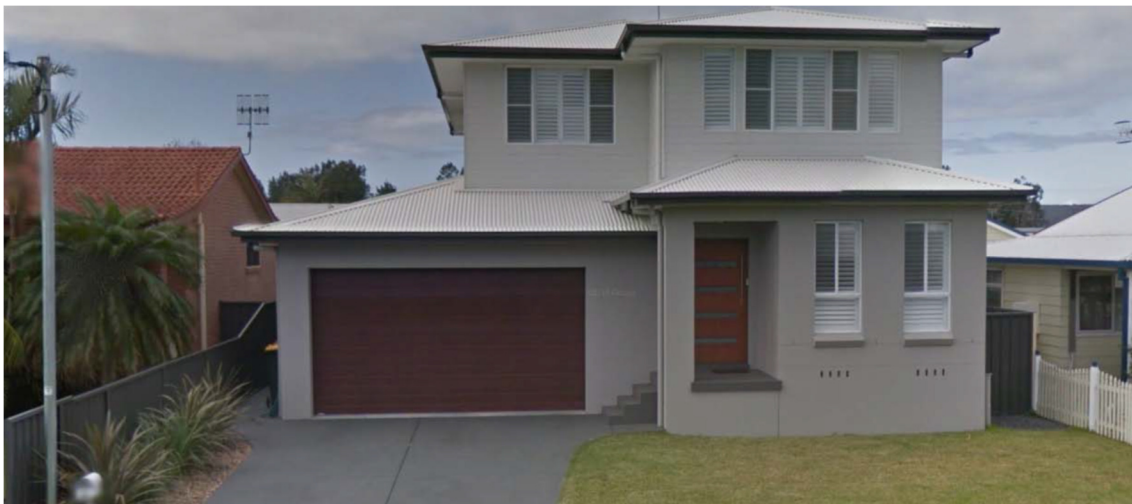
Fig11 Davistown – constructed in 2014 – FPL 2.450m AHD – floor level survey indicates a FPL of 2.042m AHD or 408mm below the required FPL
